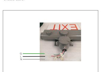
Connect the green to the grounding cable, white to null cable, black to 120V Live cable, and red to 220V Live cable.
